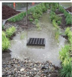
**Figure 2: Bioretention Facility**
